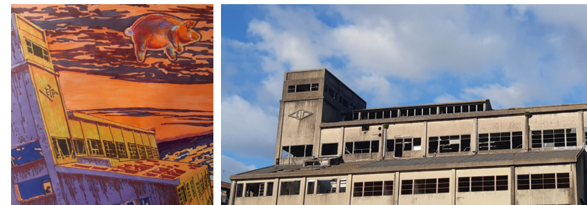
Fig. 25+26. EIF / Freixo Industrial Company | The derelict Freixo Industrial Company (EIF – Epresa Industrial do Freixo) dates from the 1940s, and is part of the land of the Power Plant, corresponding to the facilities where chemical materials resulting from energy production were recycled.
