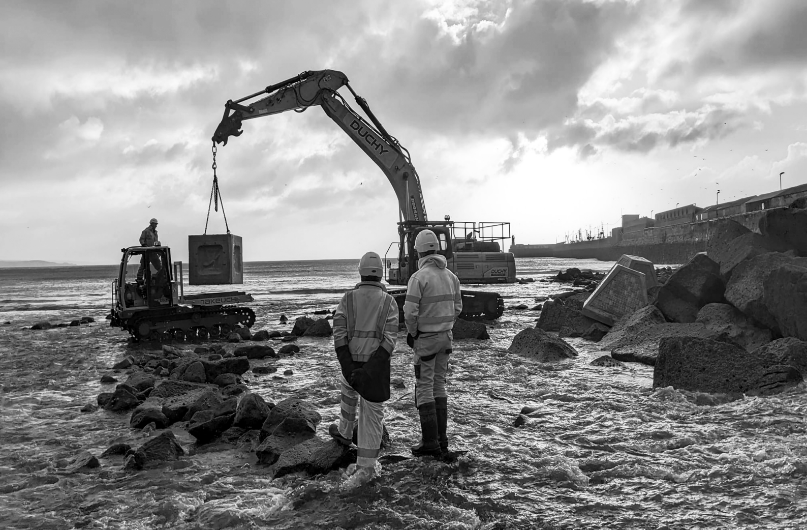
Placement of Eco-blocks along the breakwater at the Newlyn project site. Source: SARCC Project, 2022
