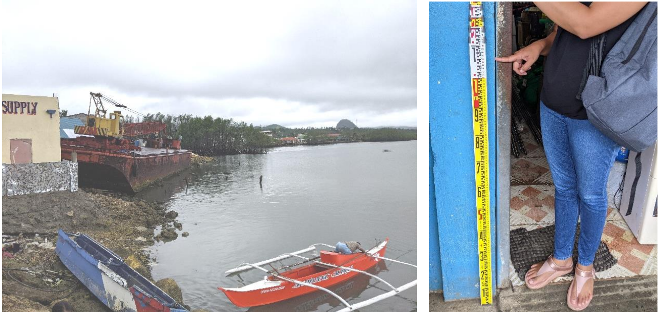
Figure 10. Left. Barge slammed into houses close to Tubigon port. Right. Inundation level in the shop seen on the left side of the figure.
