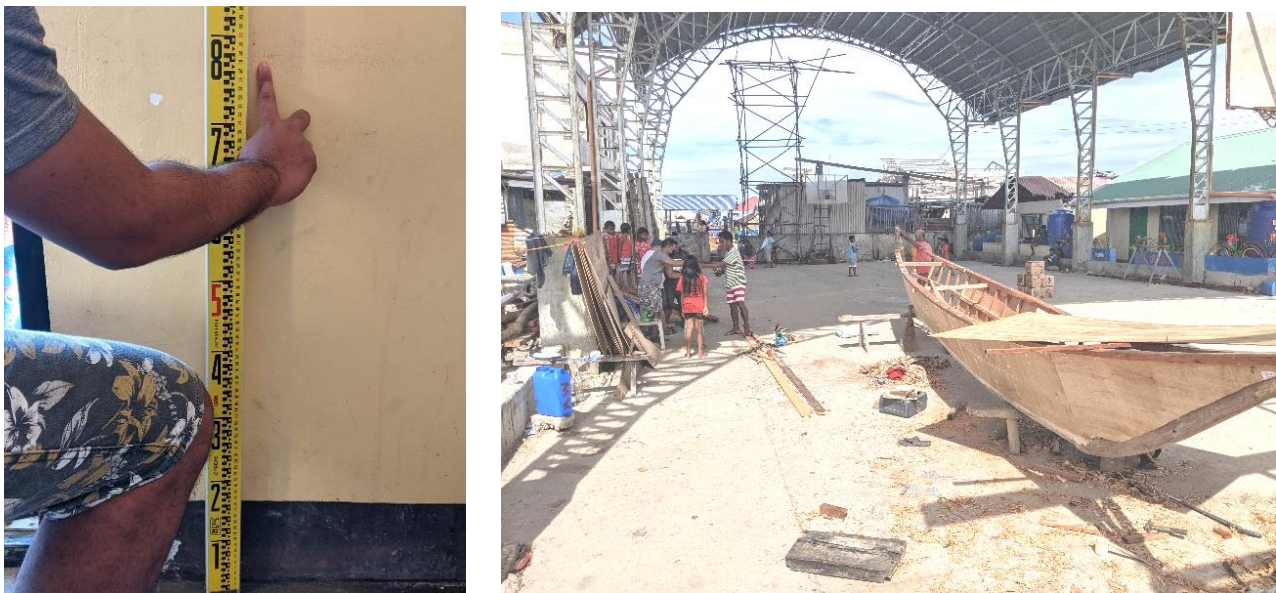
Figure 12. Left. Mudline in the barangay hall. Right. Basketball court adjacent to the barangay hall (building on the left side) and the remaining rainwater collection systems (blue cylinders on the right side).
