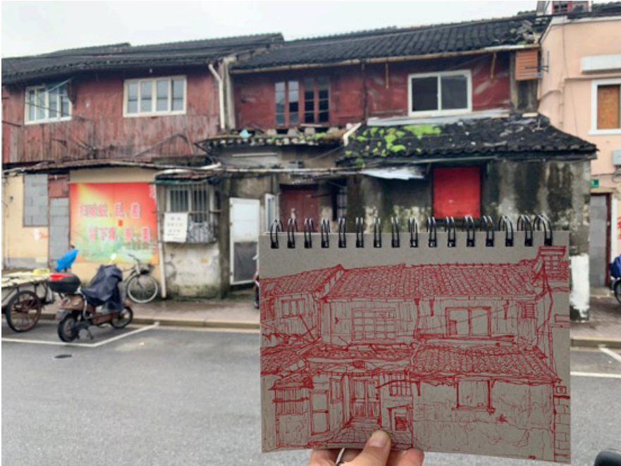
Fig. 8. Artist holding her drawing of Qiaojia Road, showing boarded-up windows and doors in anticipation of the demolition. August 2020.
