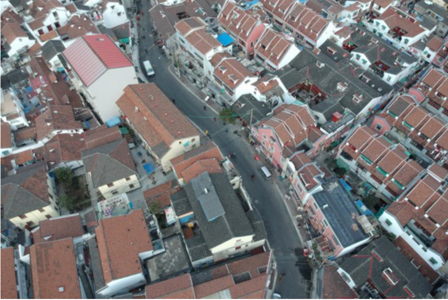
Fig. 2. Qiaojia Road, view west. On the right, Ming-era Qiao family's residence (Zuiletang) is surrounded on three sides by lilong complexes from the Republican era; Qing-era courtyard residences are seen in the distance.
