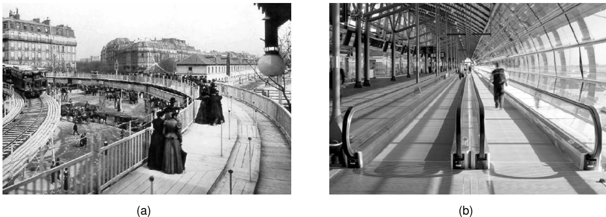
Figure 1. Moving walkways. (a) historical MW at the Exposition Universelle in Paris, 1900, composed of two parallel lanes with increasing speed. (b) modern MW installed in a transportation hub. Adapted from Avenel (1900) and Otis (2015).
