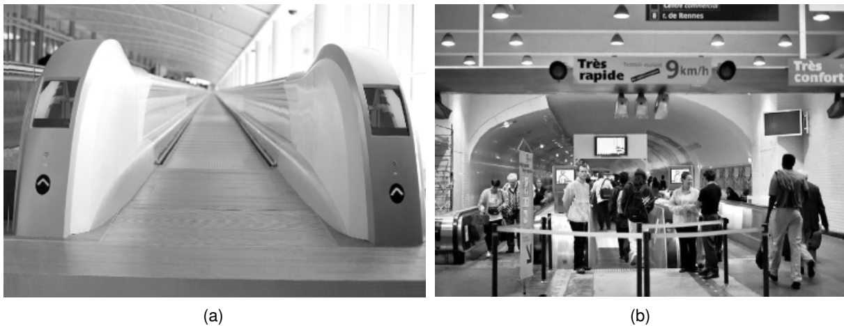
Figure 5. Accelerating moving walkway real implementations. (a) TurboTrack, Toronto airport, Canada, and (b) Gateway Paris subway, France. Adapted from Gonzalez Alemany et al. (2007), and Gautier (2000).
