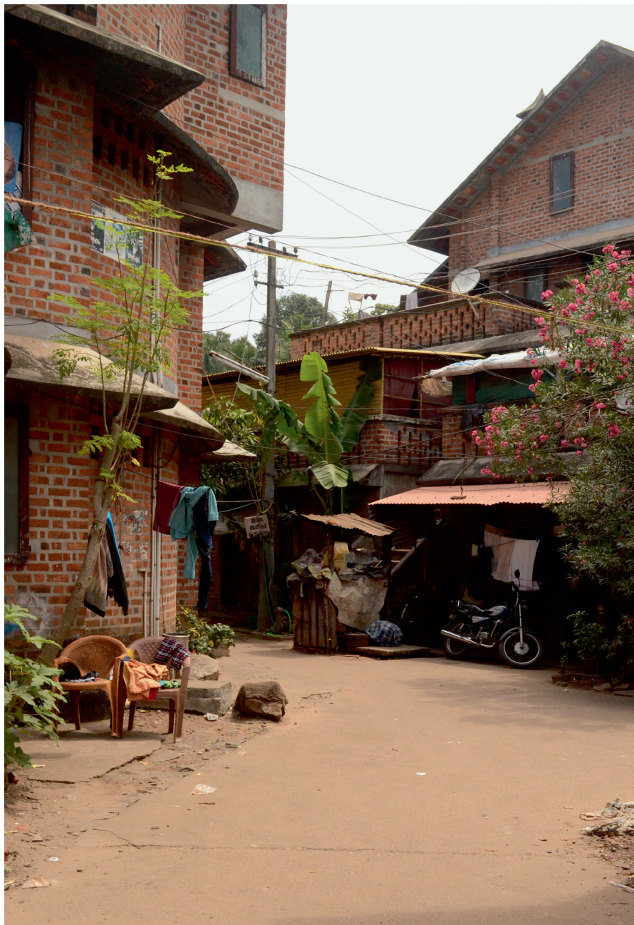
Laurie Baker, Chengalchoola Slum Development Housing, Trivandrum, foto: 2015 Laurie Baker, Chengalchoola Slum Development Housing, Trivandrum, photo: 2015
