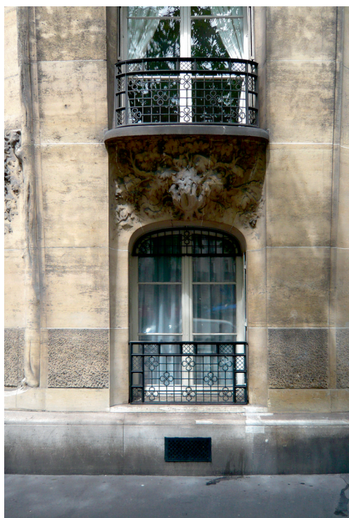
Geveldetail met ornament Detail of façade with ornament
