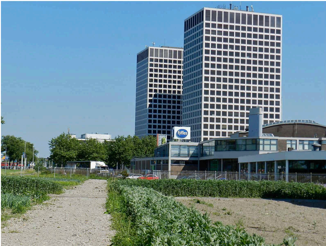
FIGURE 5.5 The 'Uit je Eigen Stad' (From your own city) Foundation initiated the city farm Marconi-strip. This former marshalling area in the Merwehaven in the City Ports is a temporary farm before it will be developed into a mixed residential/work area. The foundation aims to bring the food back to people in the city; it also links government, education, business, and science. The project also provides workspace for participants in reintegration programs (image courtesy of Kees van Oorschot)
